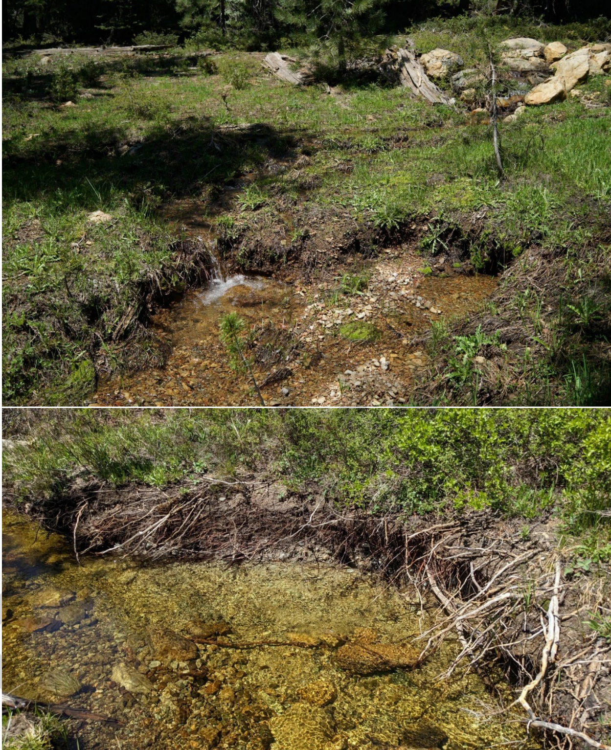
Figure 11. Areas of poor meadow surface hydrology in Mumbo Basin, showing a headcut feature (top) and incised banks (bottom). Similar signs of degradation are fairly common throughout the assessment area, and offer opportunities for small-scale projects to expand and enhance wet meadow habitat.
