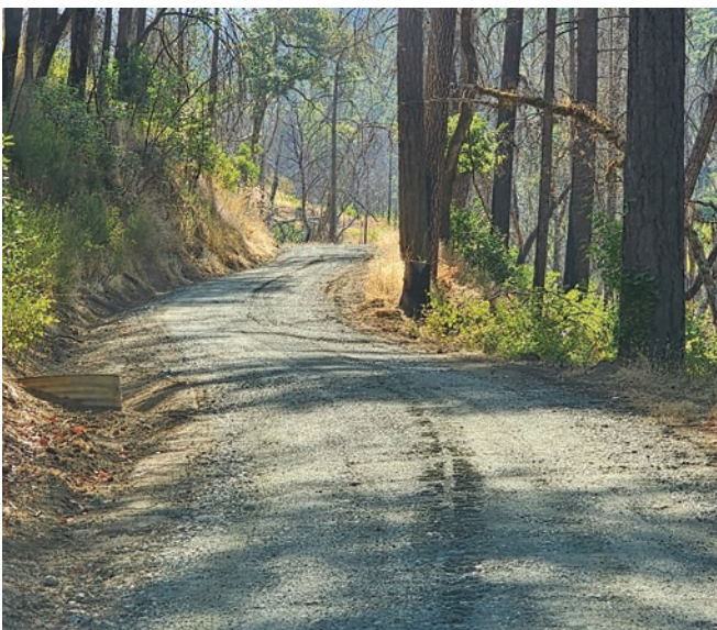
Bordy Creek Road in Big Bar. Inboard ditches were cleaned, rock rolling dips reconstructed, and the road shaped and rocked
