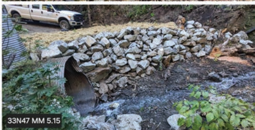
Woody debris and a damaged inlet threatened the road crossing in Soldier Creek. Damaged sections of culvert and logs were removed, and the streambank was armored with rip rap
