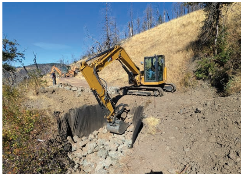
100% plugged culvert caused a partial washout of this stream crossing; rock armoring was added until the culvert can be replaced with a larger diameter one. Eel River watershed
