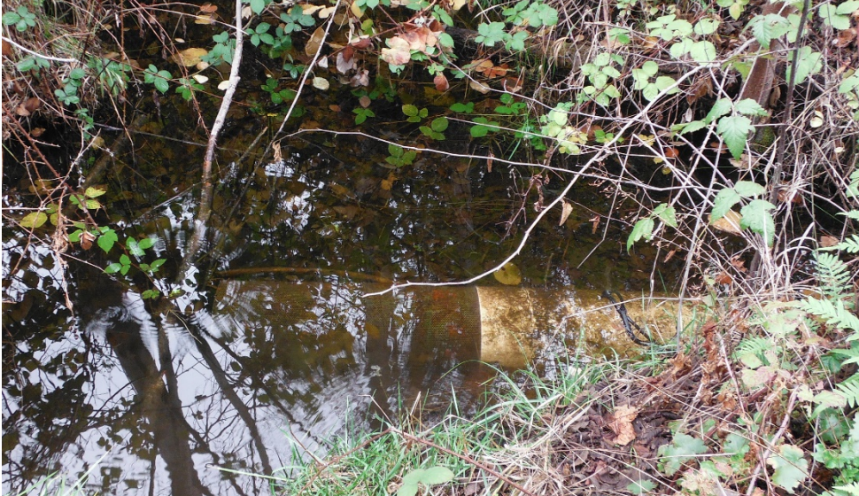
Figure 6. Diversion tube intake with fish screen at Olsen Creek.
