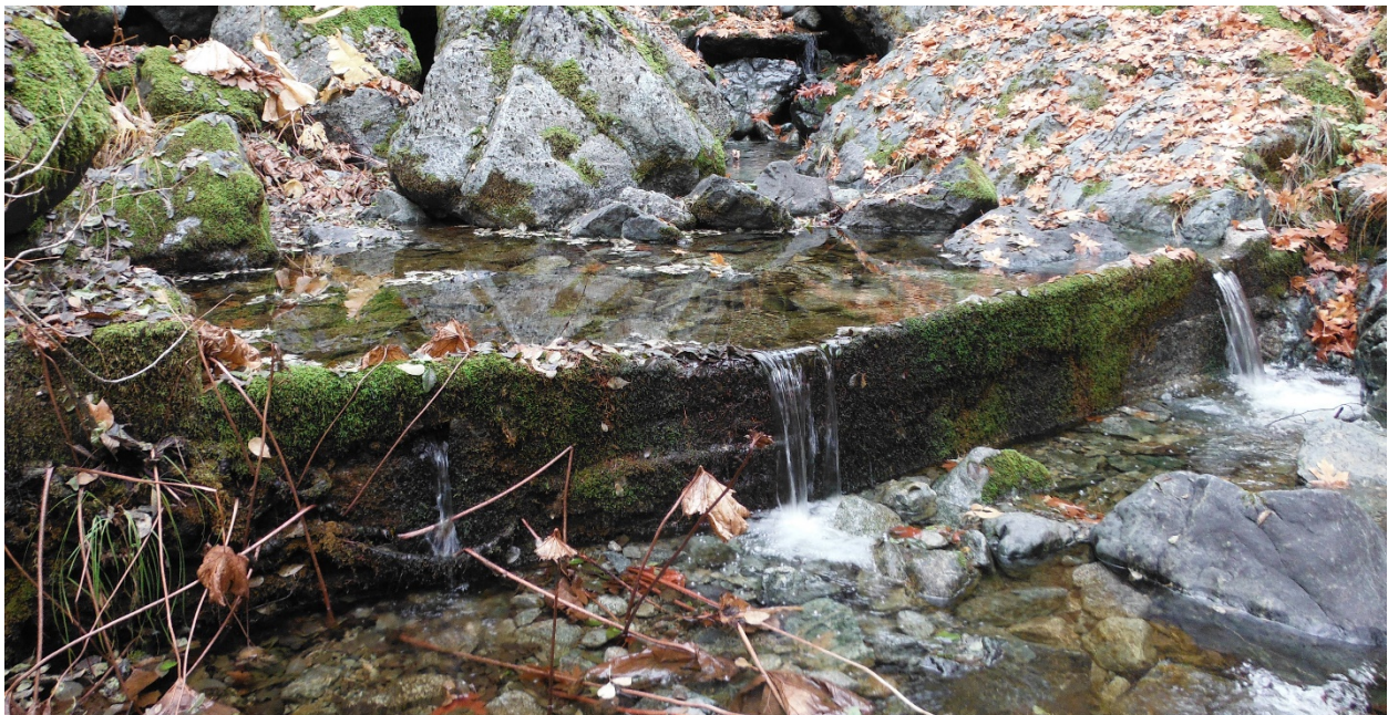
Figure 8. The diversion dam at Silver Creek.
