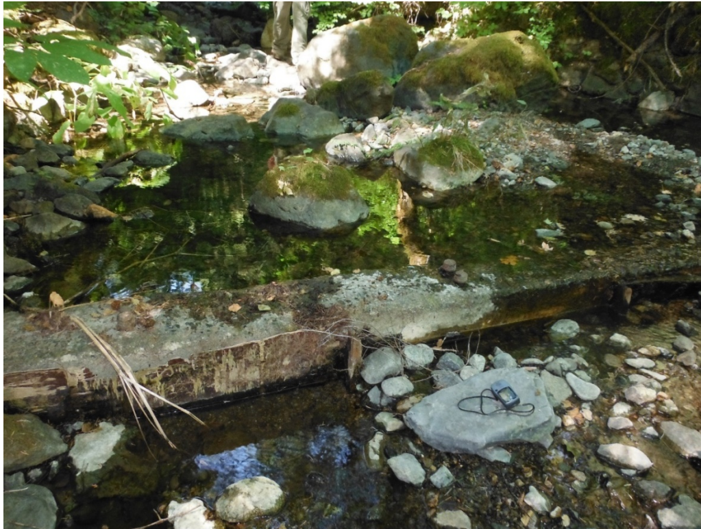
Figure 14. The diversion on West Tule Creek.
