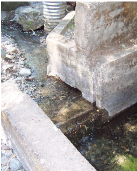
Figure 10. Big Creek upper diversion flows over diversion structure (a) and into the fish passage structure (b).
