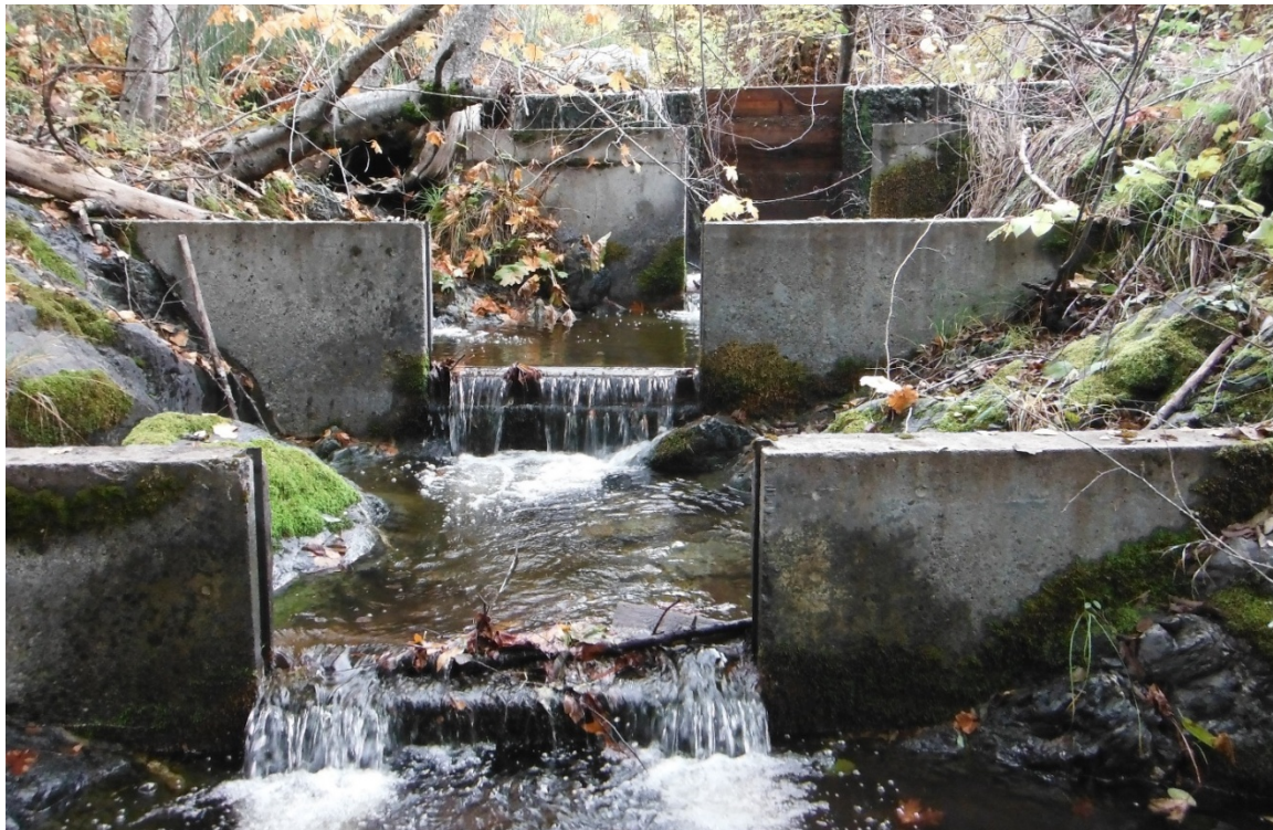
Figure 7. Fish passage structure at Olsen Creek.
