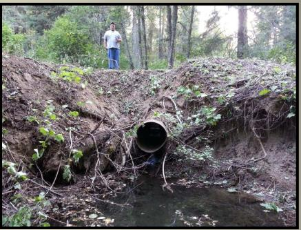
This photo taken just before we excavated the culvert, site has been grubbed of vegetation. You can see where water has went over the road at times and can see the shotgunned culvert which was a fish barrier to resident Steelhead.
