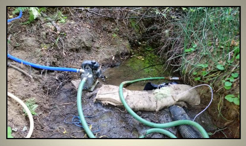
Diverted creek via 6" plastic flex pipe, with small sandbag gravity flow diversion dam, we did partial excavation and then later we plugged flex pipe and used pump to take water around second half of excavation.
