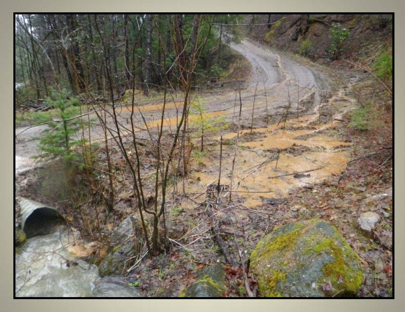
Disconnect ditches and road surface erosion from streams
