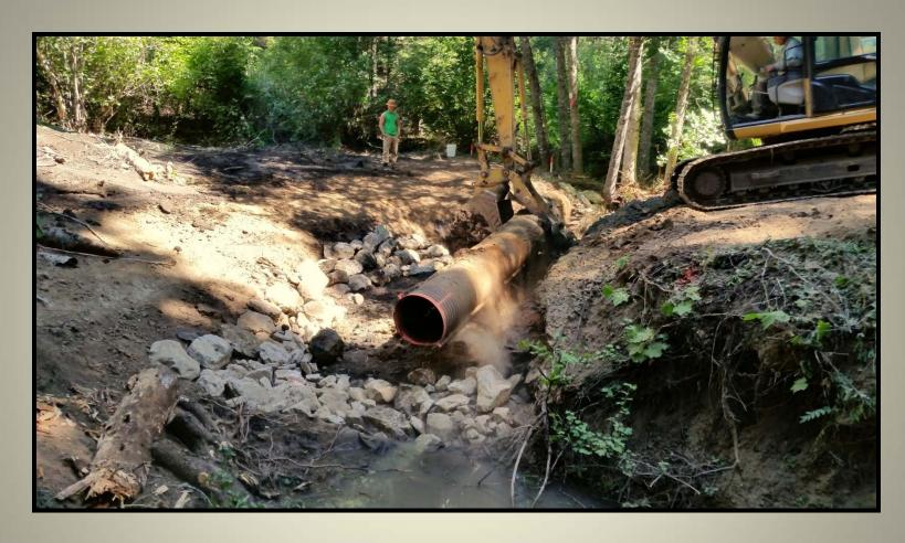
At the time we pulled the culvert, the creek was being diverted (pumped) around the site entering below our construction area.
