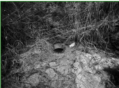
*Without a sediment riser a culvert can easily get plugged with accumulated sediment.*
