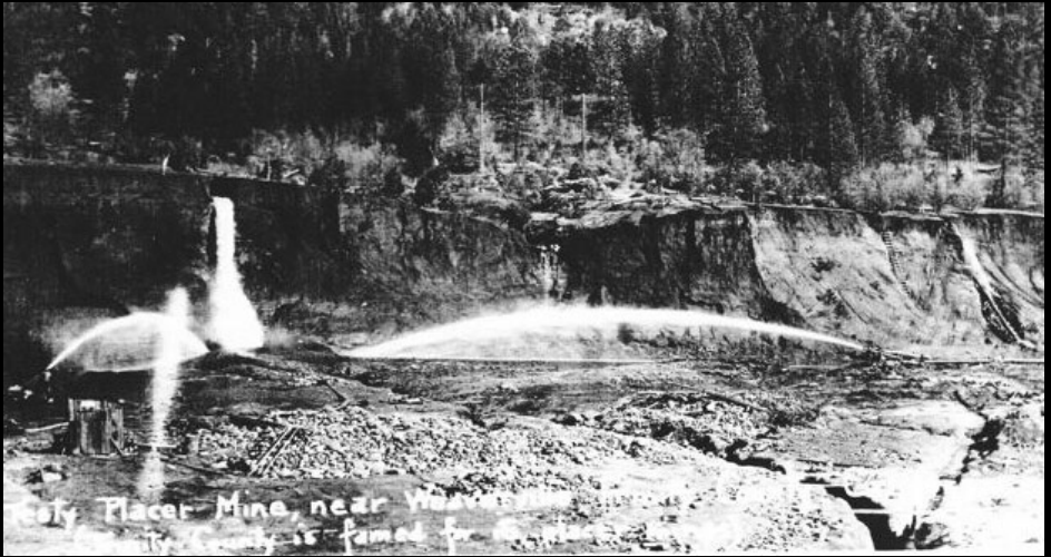
The Testy Placer Mine near Weaverville
