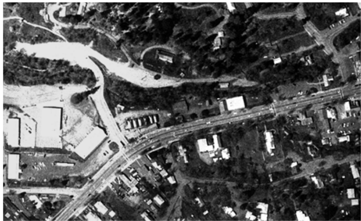
Aerial photograph of the Trinity Gateway site.
