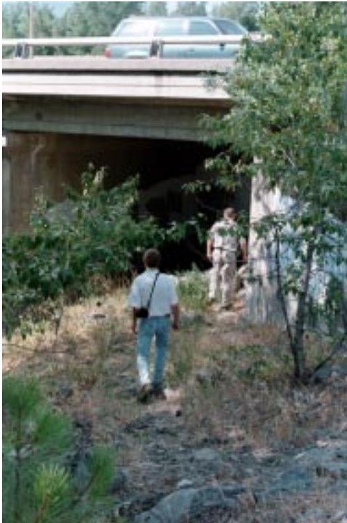
Photograph #6 -- Existing View of Highway 299 overpass.
