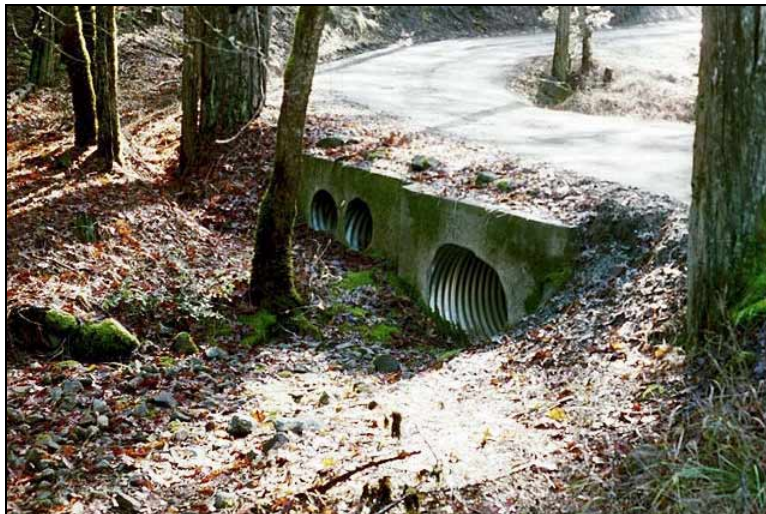
Culvert installation
