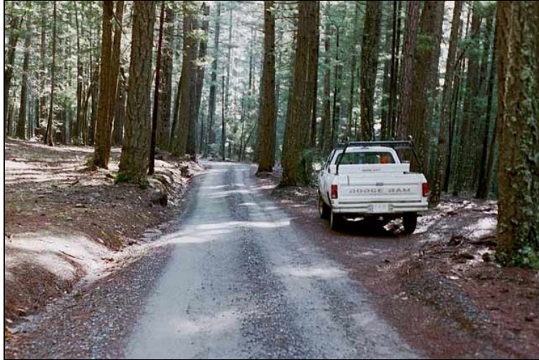
Constructed turnout
