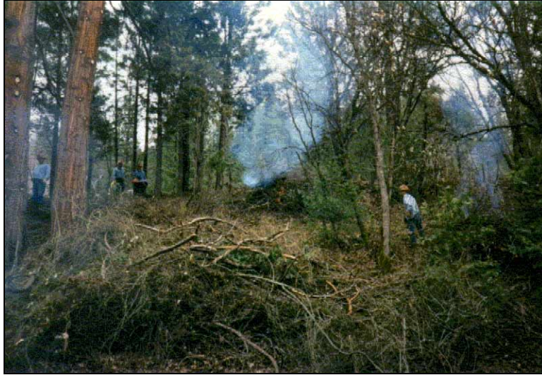
Fuel Reduction Work along East Branch
