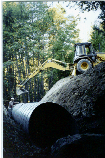
Installation of Upgraded Culvert
