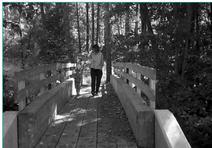
New Bridge Over East Weaver Creek
