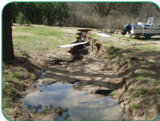
Chandler Pipe Upgrade-Before
