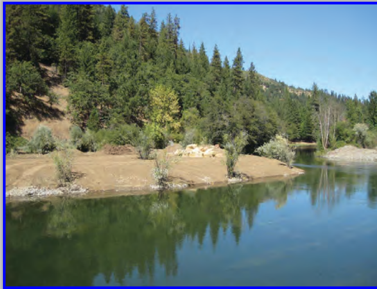
Newly constructed forced meander; previously the river traveled in a straight line, now has a significant bend.
