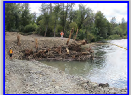
Habitat structure completed
