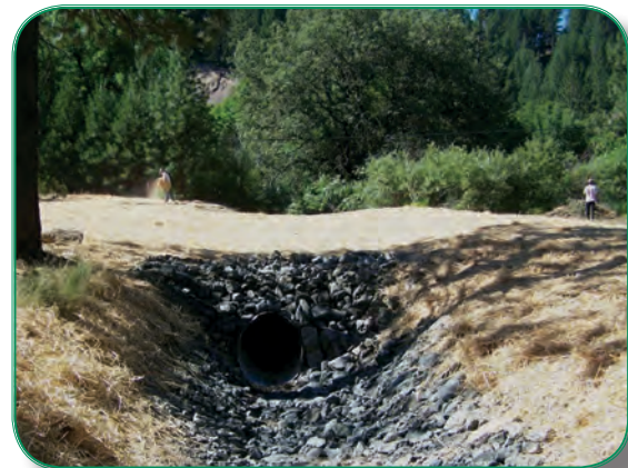
Chandler Pipe Upgrade-After
