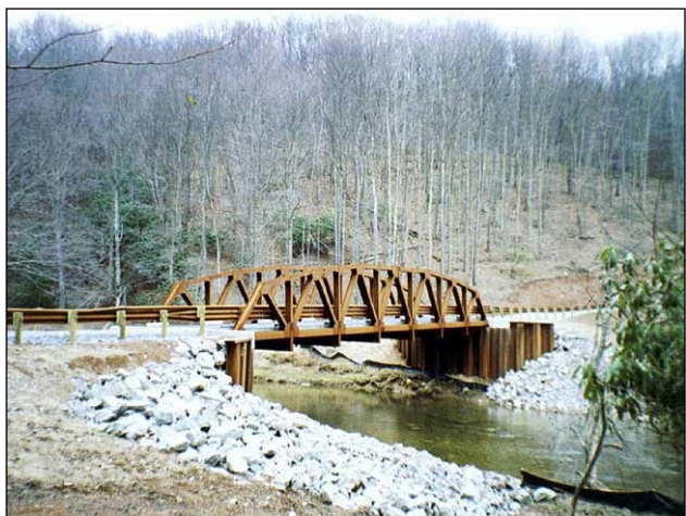
Example of Steel Truss Replacement Bridge
